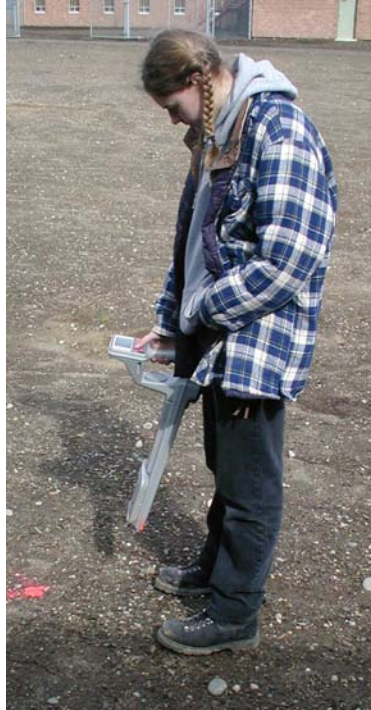
Figure 7 - Tracing a Pipe
